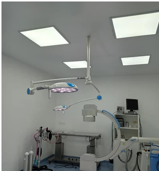
Figura 6: Infraestructura Hospitalaria IEES (Latacunga)
