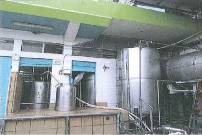
A photograph of an industrial area, likely for milk reception. It shows several large, vertical stainless steel storage tanks or processing units. A network of pipes and valves is visible, connecting the tanks. The area is well-lit, and the ceiling has a green-painted beam. The overall environment appears clean and organized for industrial operations.                                          |
