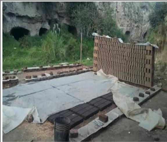
**Fotografía 2.** Oreado de los ladrillos
