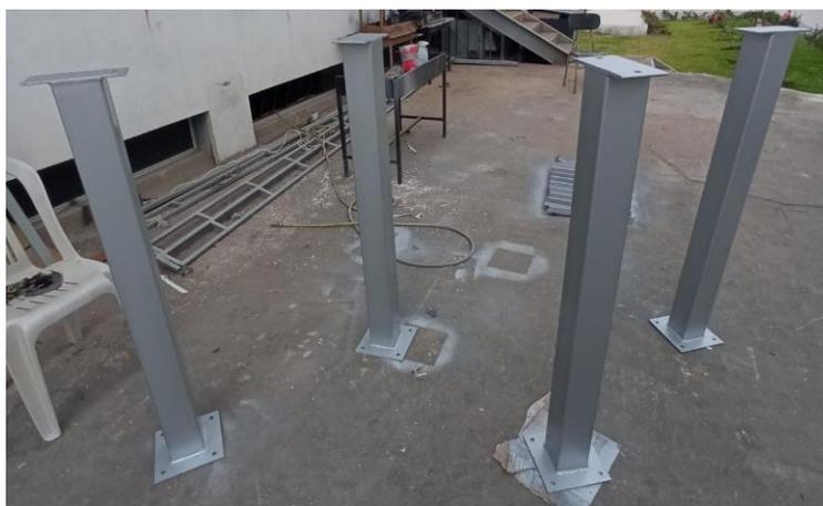
**Figura 5.21.** Bases desmontables
