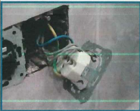
Plug with taking of earth (yellow and green wire)
