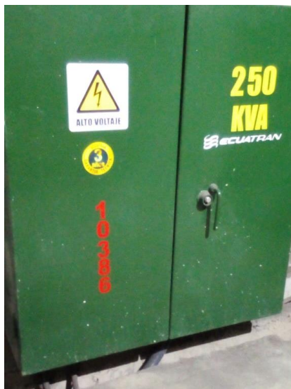
Figura 4.4. Transformador Pad Mounted Trifásico de 250 kVA,13.8 kV/220-127 V.
