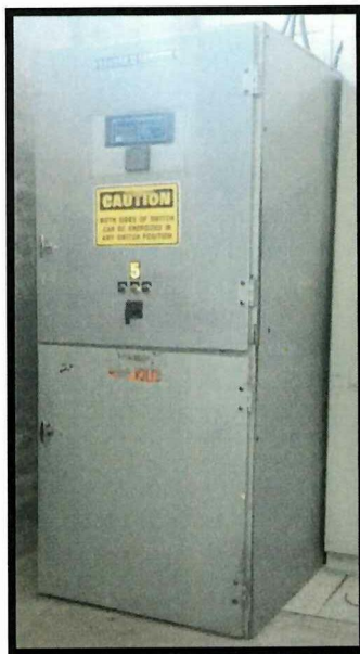
Figura No. 3.7 Interruptor Disyuntor
