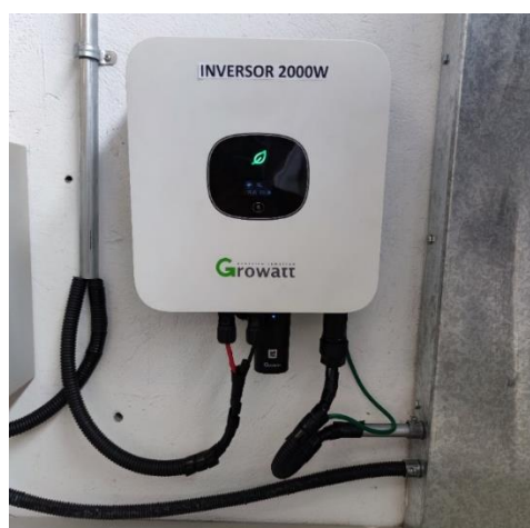
Figura 39. Inversor ON GRID Growatt de 2000W.
